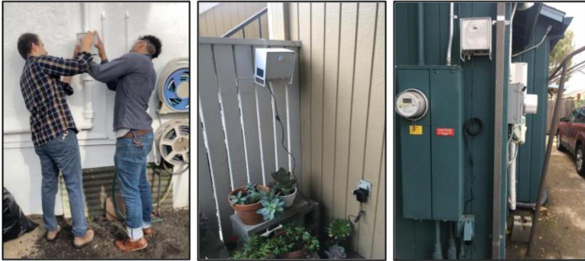
**Figure 15. Examples of Aeroqual AQY 1 micro air quality monitor deployment in Richmond-San Pablo.**
