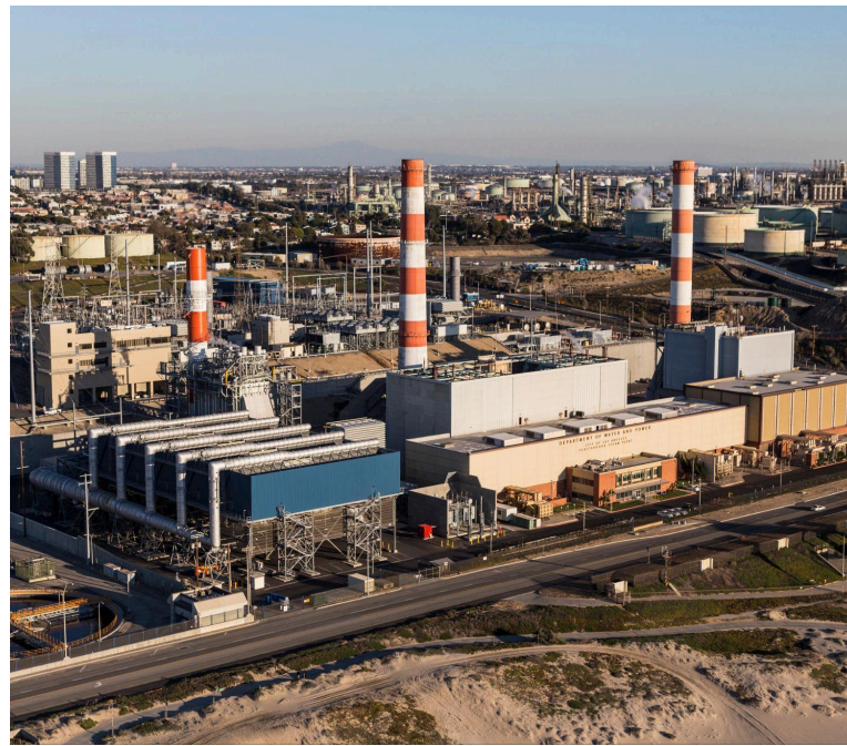
Scattergood Generating Station, Los Angeles
